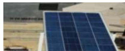
Fig. 12 Panel Solar ERDM 135SP6 de 135W a 20V
