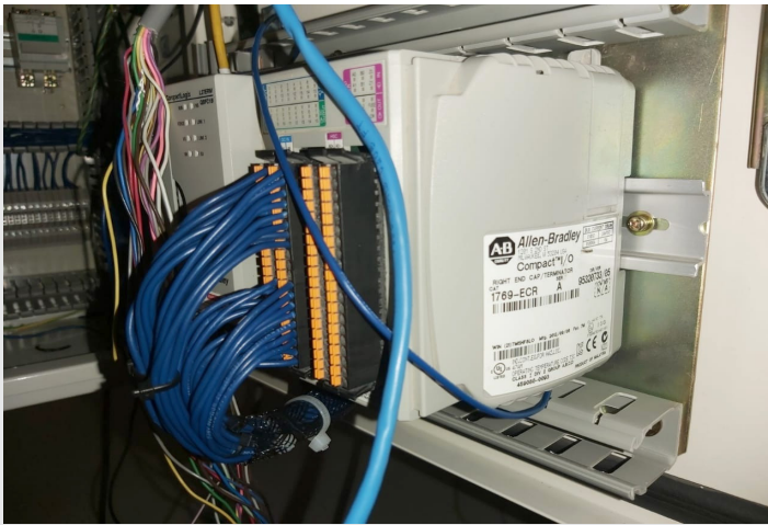
Figura 3. PLC Allen Bradley 1769.
